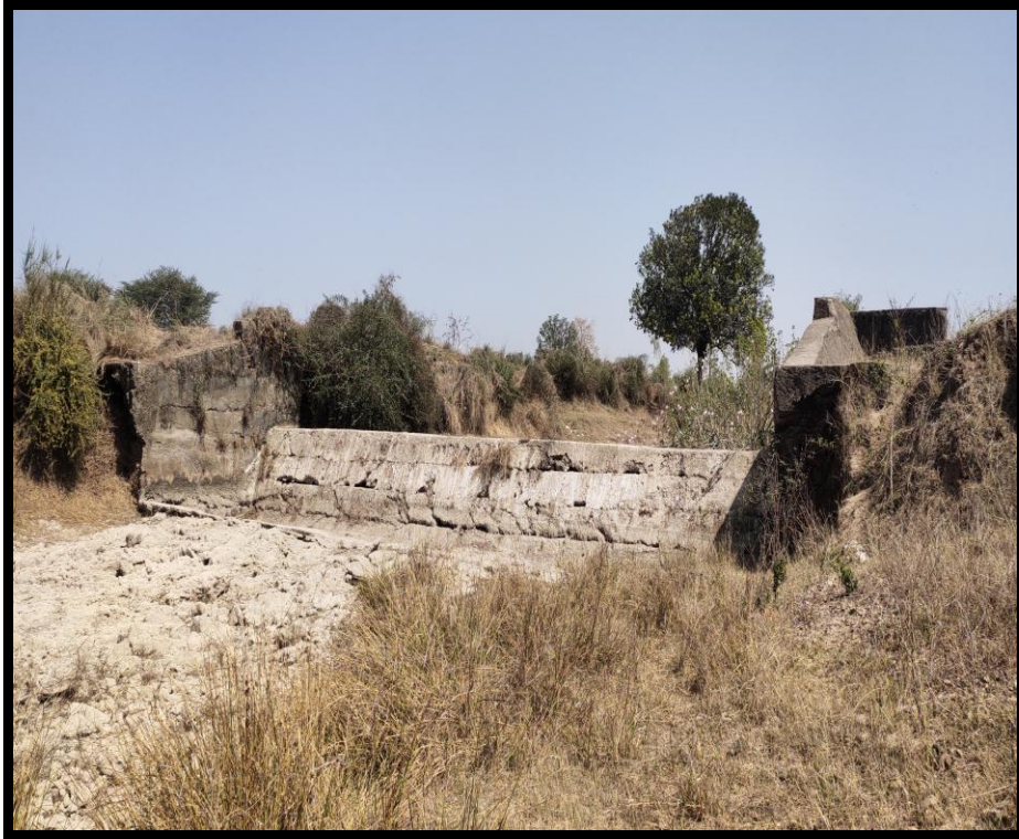
HFL on Check Dam
